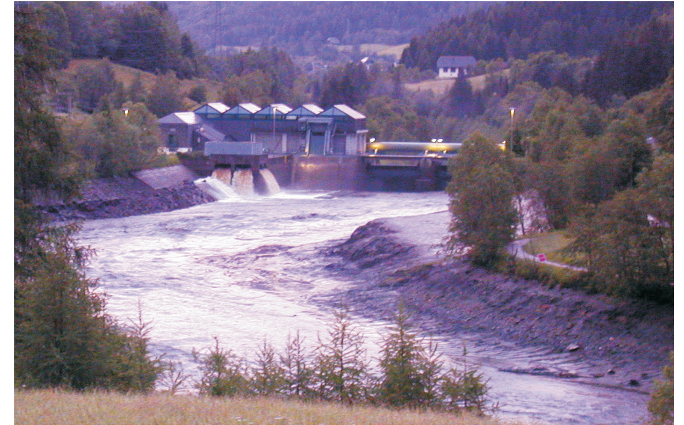
Power plant Bodendorf during the flushing
