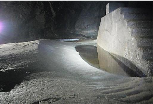
Fig. 6 Prototype sand accumulation before rake to pressure shaft ( [2])
