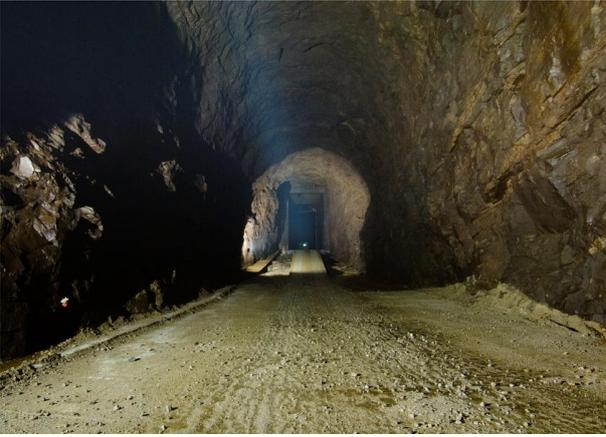
Fig. 4 Unlined pressurized sand trap, view direction upstream
