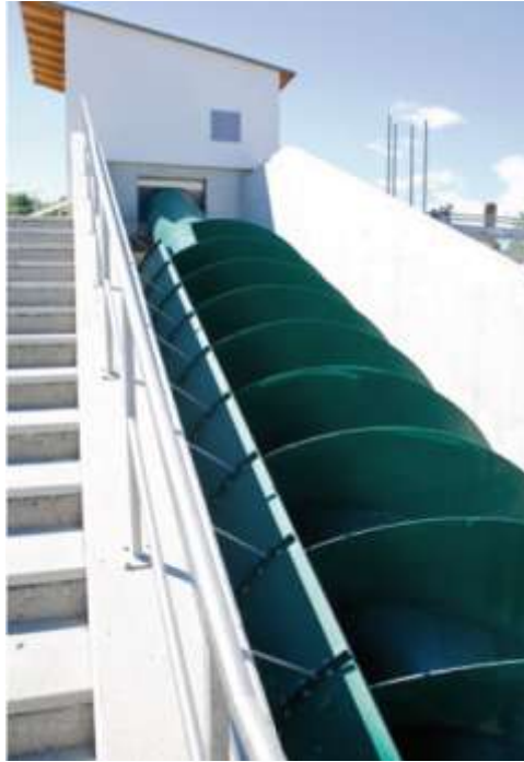
Figure 34: One of the hydrodynamic screws at Niklasdorf power plant ( BEA Electrics )
