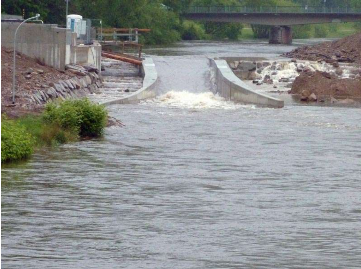
Figure 12: Power plant Gengenbach (source: http://www.moveable-hepp.com/ )
