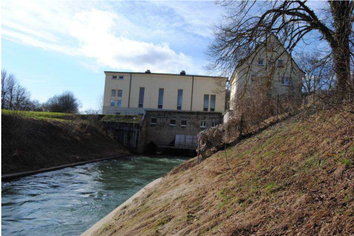
Figure 38: Main power house of HPP Rappenberghalde, view from tailrace channel (photo [Renz, 2011])
