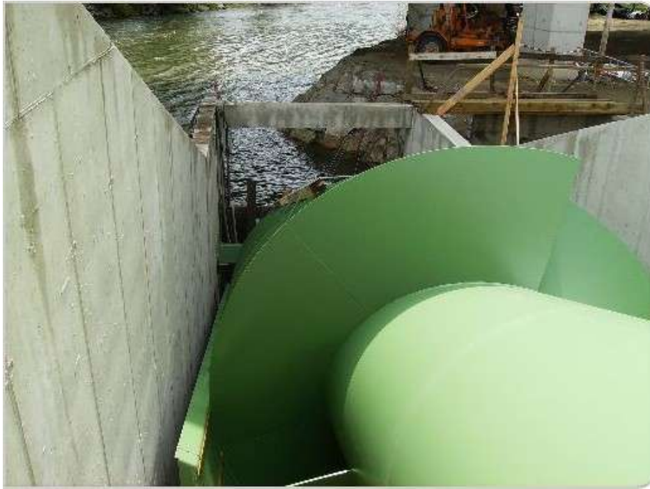
Figure 31: Detailed view of hydrodynamic screw (Schalungsbau Hager Ges.m.b.H.)
