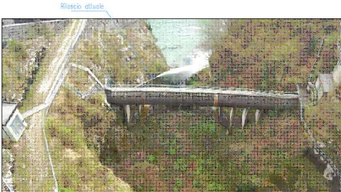
Figure 14: Present Mis' dam situation. The light blue arrow indicates the present MIF release
