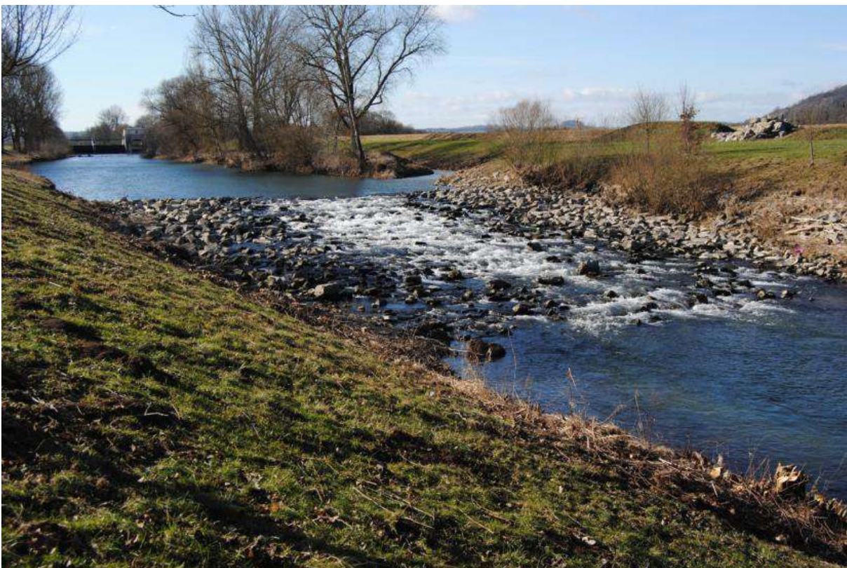
Figure 41: New rock ramp instead of concrete weir in diversion reach (photo [Renz, 2011])
