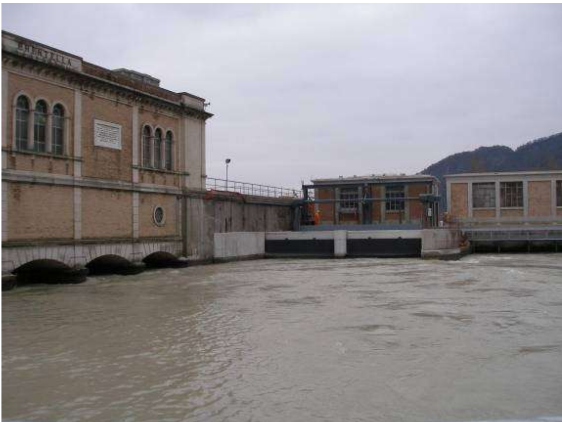
Figure 20: The power plant completed (upstream point of view)
