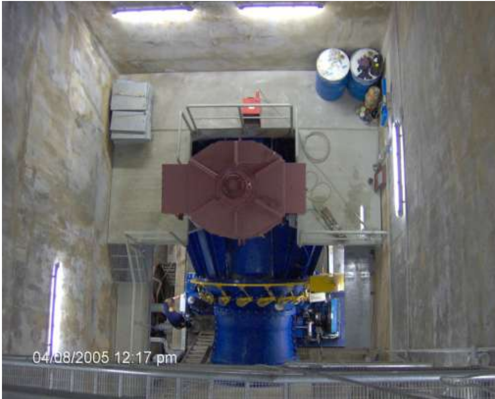
Figure 24: Busche power plant machine (horizontal axis Kaplan)
