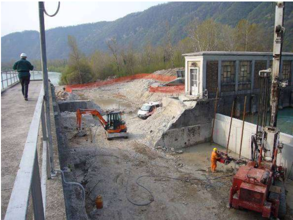
Figure 18: The beginning of the construction works
