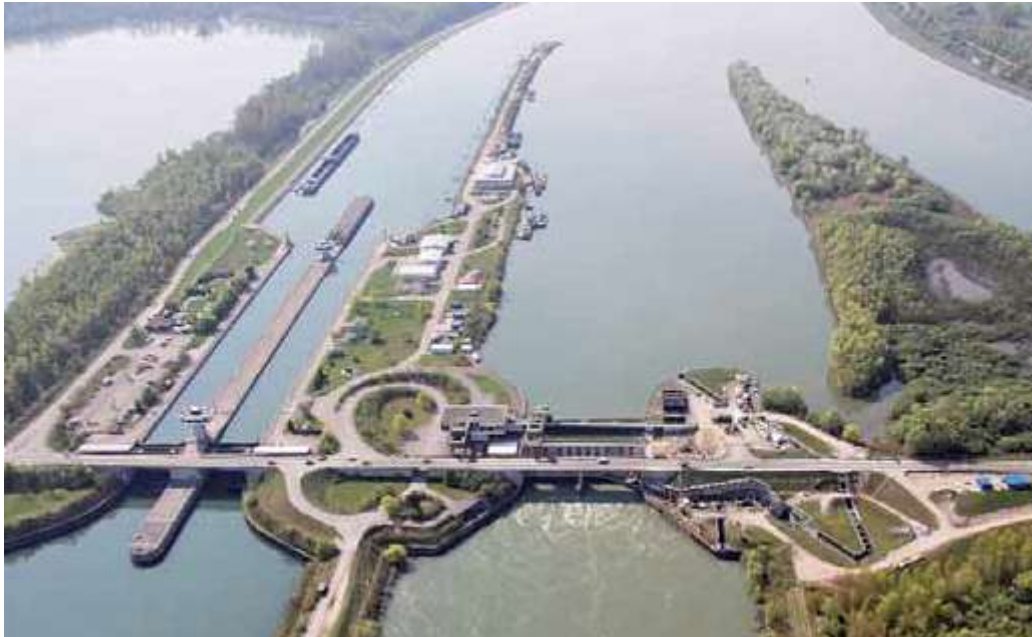
Figure 42: Iffezheim barrage on Rhine, view of a double ship lock, a power house and a new fish pass. Photo (EnBW, 2009)
