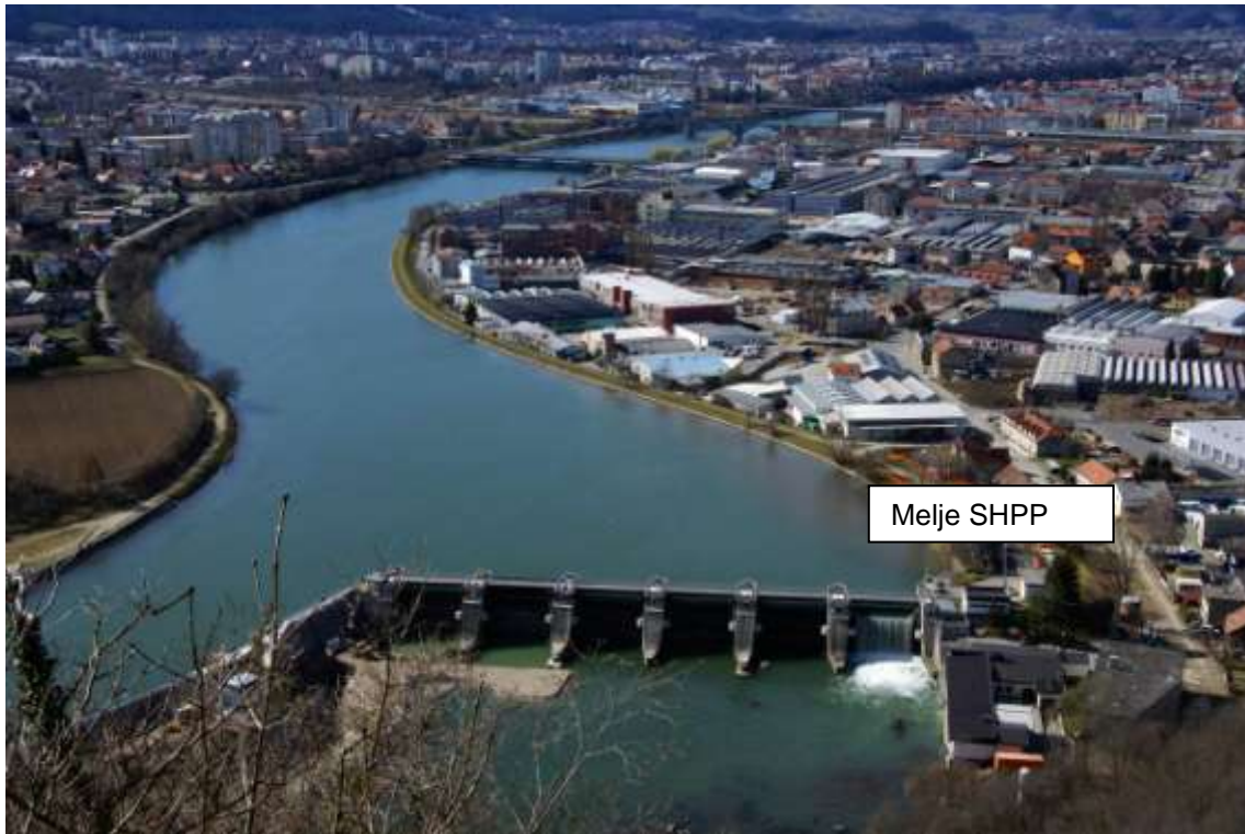
Figure 26: Melje Dam with assigned location of Melje SHPP
