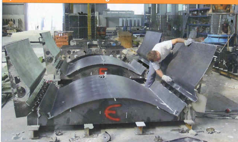
Figure 10. Special moulds for ribbed segments.
